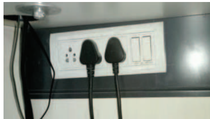
8 Module Switch Plate with 3 sockets and 2 switches
